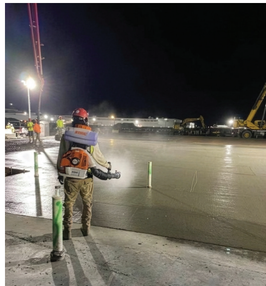
Fig. 1: Early fogging is necessary to maintain the reflective appearance of the damp concrete. With the changing nature of Type II cement, contractors need to consider environmental factors and keep concrete surfaces continuously damp, without allowing water to accumulate (photo courtesy of Ben Wiese)
